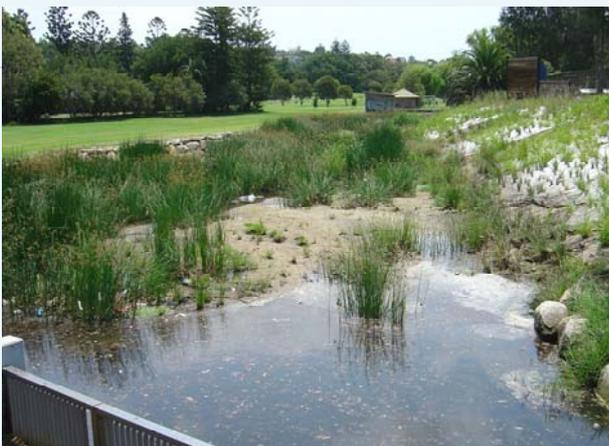
Stormwater then flows into a small wetland that helps to remove nutrients from the stormwater runoff before it flows to Rose Bay.
