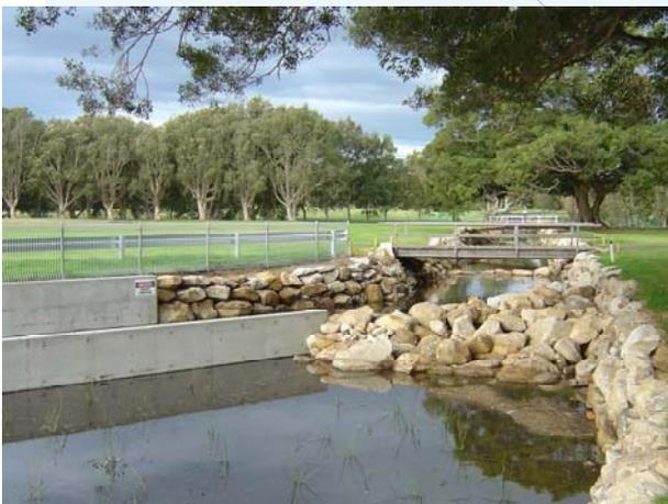
The upstream crumbling concrete walls were replaced with sandstone and vegetation to provide habitat for birds and reptiles, and to improve stormwater quality.
