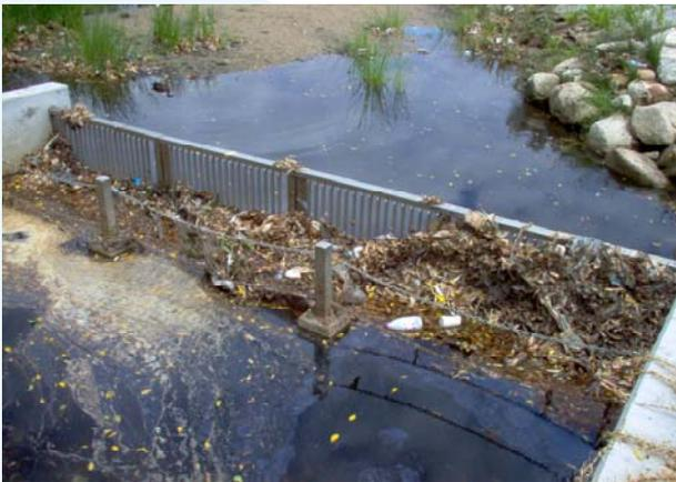
A trash rack is also used to capture gross pollutants, such as litter and grass clippings.
