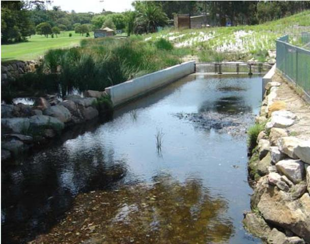
Stormwater flows down the 'naturalised channel' into the sediment trap, which captures sediments.
