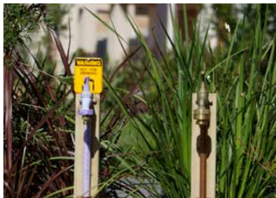
Recycled water garden taps have a removable handle and need to have a warning sign near them.
