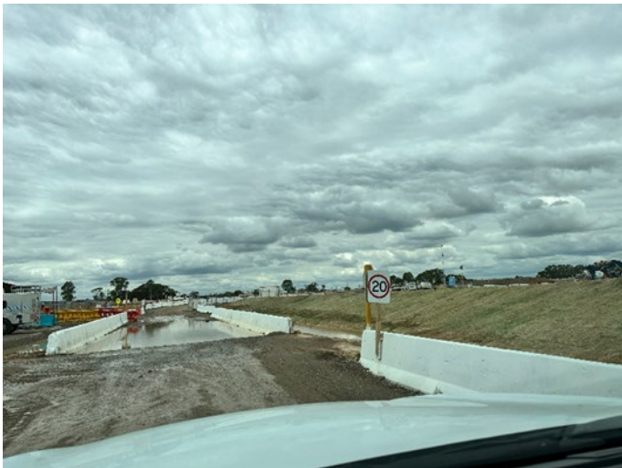
Photo 11: Speed restriction signage and wheel wash - AWRC site
