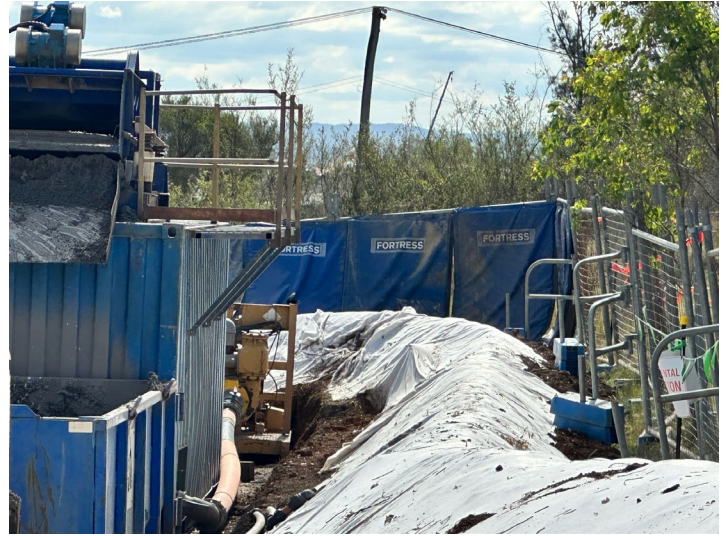
Photo 28: Acoustic blankets (HDD operations)– treated water pipeline
