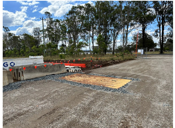
Photo 14: Stabilised site access – treated water pipeline compound site
