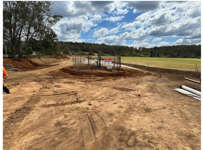
Photo 6: HDD retrieval pit - treated water pipeline
