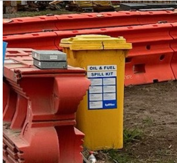
Photo 32: Oil and fuel spill kit – AWRC site
