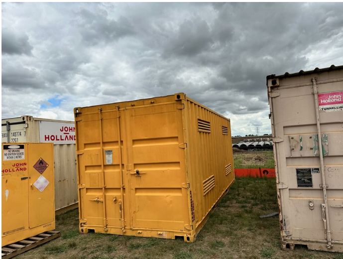
Photo 29: Chemical storage container – bunded and ventilated
