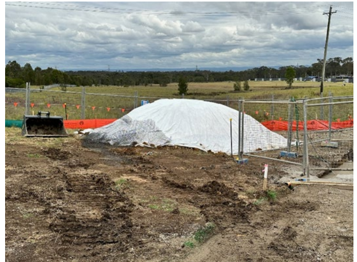
Photo 10: Temporary Stockpile covered – AWRC Site
