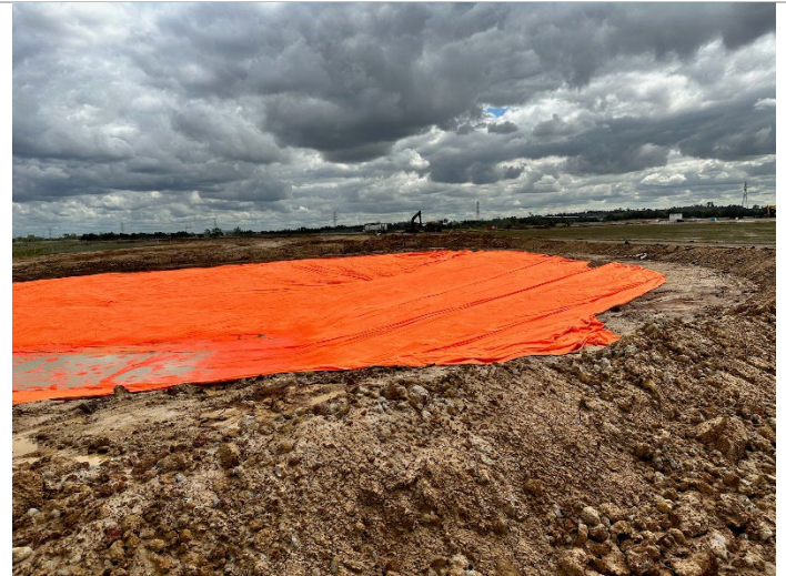
Photo 18: high efficiency sediment basin under construction – AWRC site
