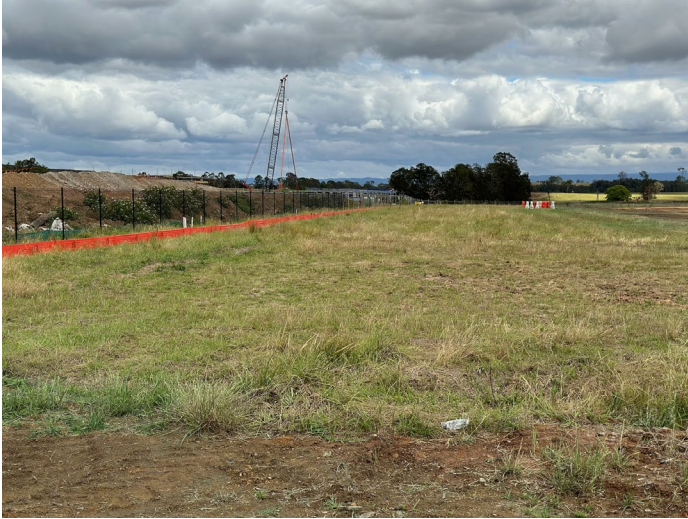
Photo 17: groundcover and sediment fence – AWRC site
