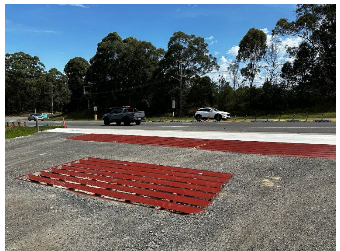
Photo 10: Hardstand site entry/egress and rumble grid
