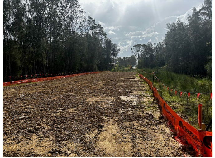
Photo 34: Sediment fence and boundary fencing
