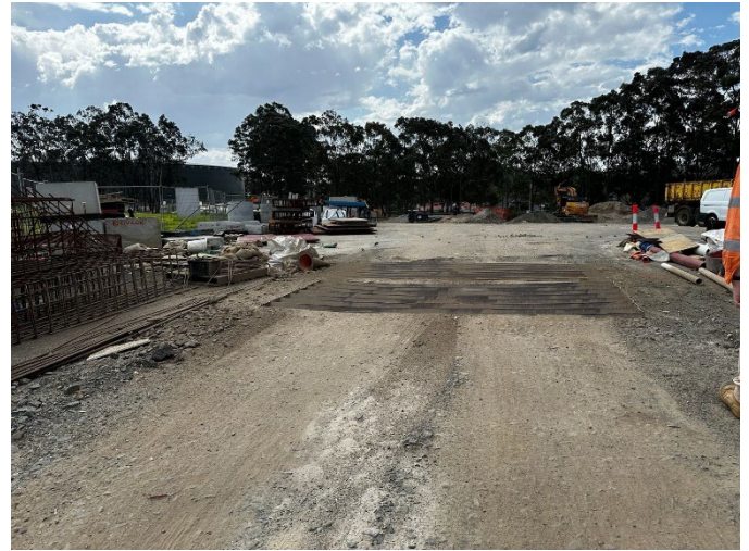
Photo 2: Stabilised access with rumble grid
