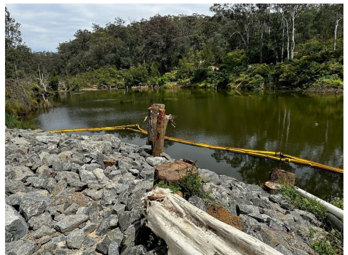
Photo 26: Silt curtain/oil boom – Nepean River
