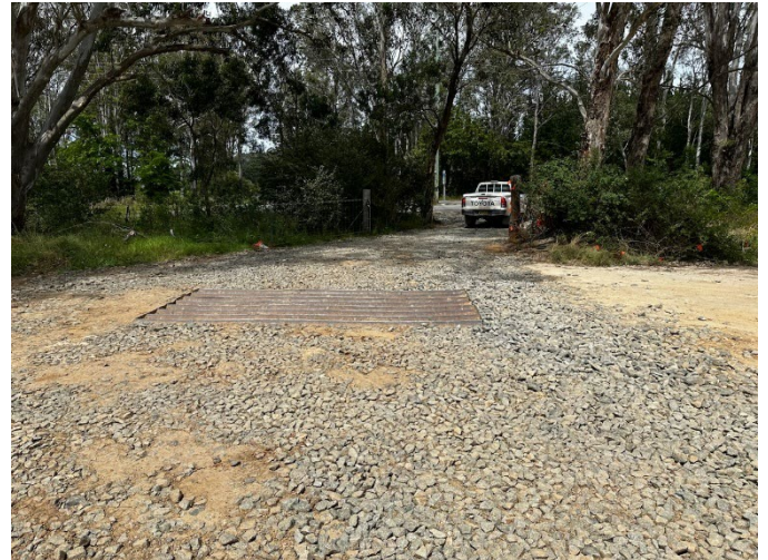
Photo 30: Stabilised site access/egress and rumble grid
