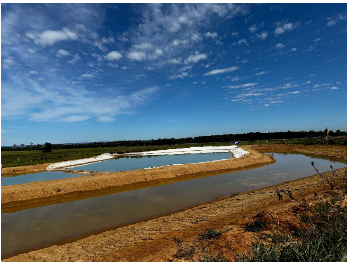
Photo 37: High Efficiency Sediment Basin
