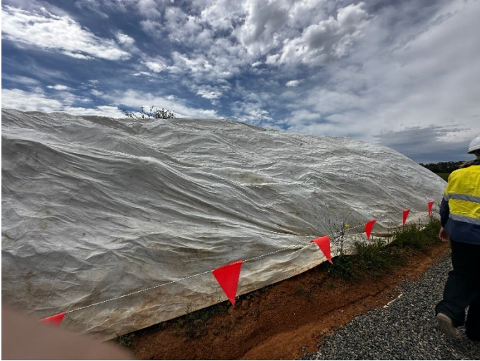
Photo 27: Geofabric covered stockpile
