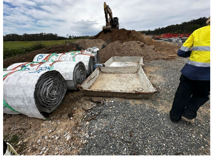
Photo 28: Waste concrete washout trays
