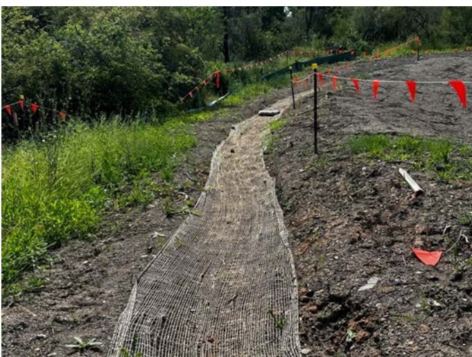
Photo 9: Jute mesh lined drain
