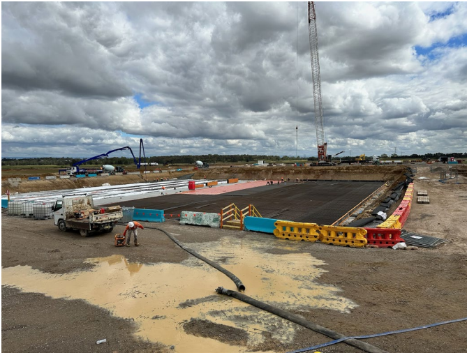
Photo 1: General construction works – AWRC site
