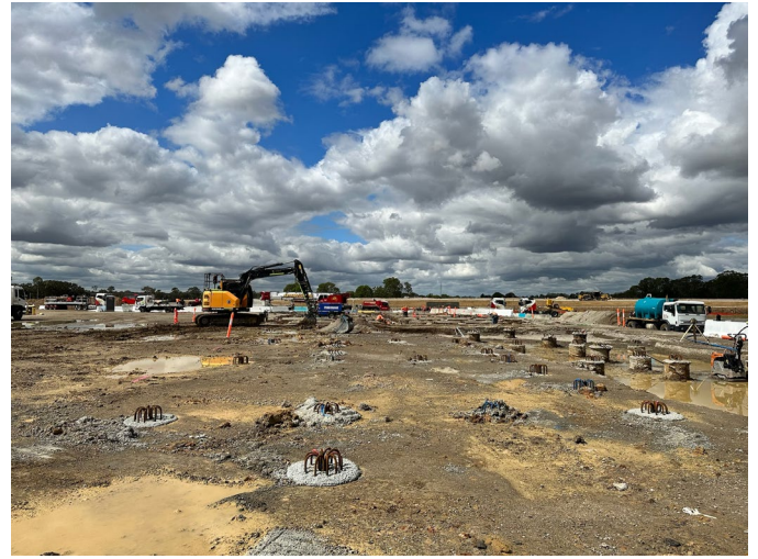
Photo 2: Piling and ground engineering – AWRC site
