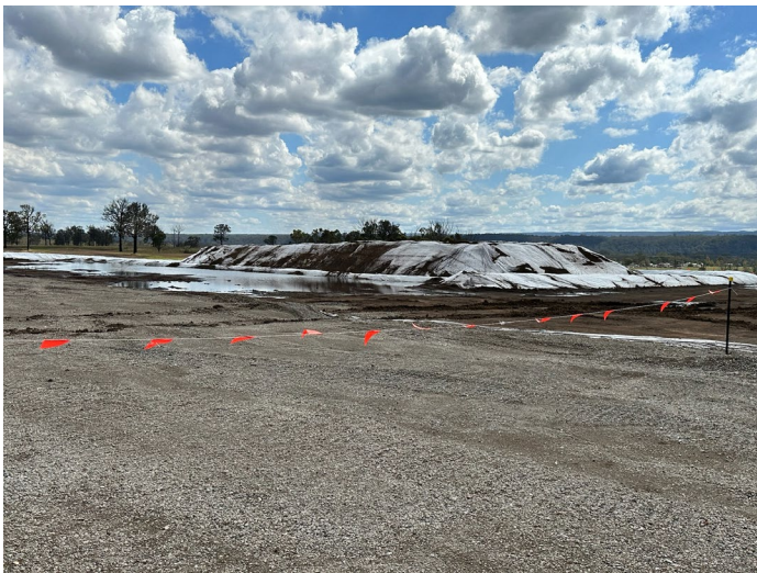
Photo 15: Spoil stockpile covered with geofabric - treated water pipeline compound site
