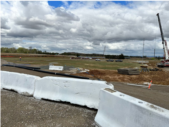
Photo 3: Soil stabilisation and rehabilitation work – AWRC site
