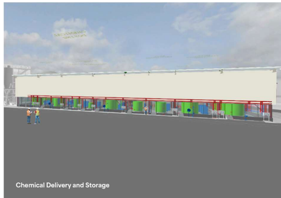
Figure 97 Preliminary design studies for cladding on Chemical Storage building to reduce solar absorptive criteria
