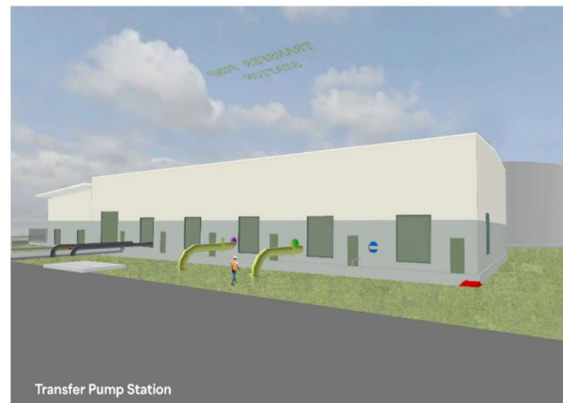
Figure 100 Preliminary design studies for cladding on Transfer Pump Station building to reduce solar absorptive criteria
