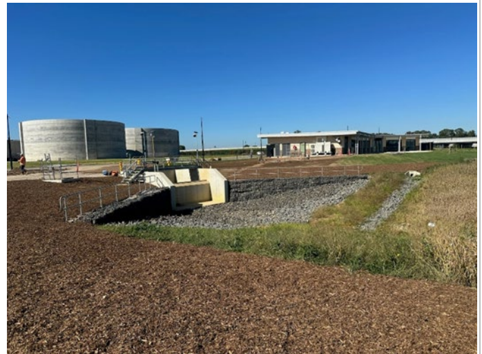
Photo 4: AWRC Outlet, Administration building and brine tanks
