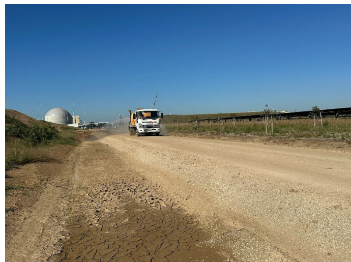
Photo 16: Streetsweeper Water Cart utilised for dust suppression
