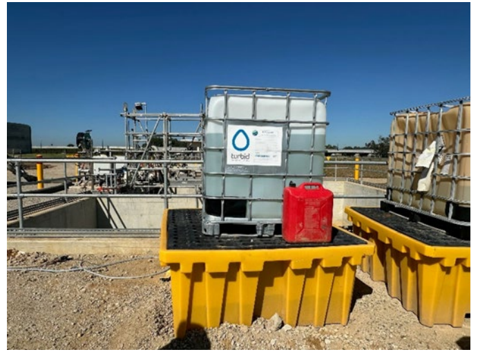
Photo 18: Chemicals stored in mobile bund
