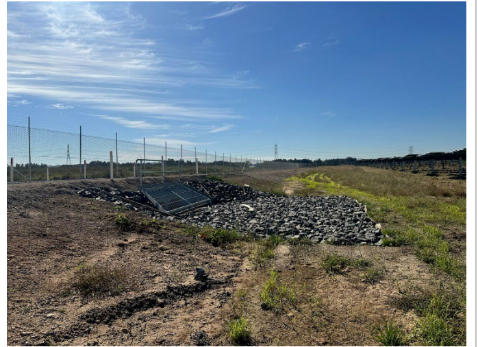
Photo 8: Permanent drainage and culvert adjacent to the Solar Farm
