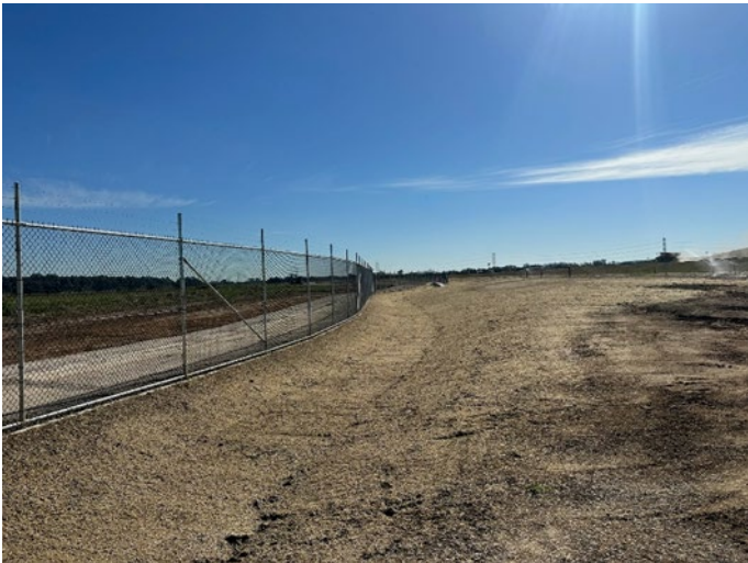
Photo 11: Permanent fencing and stabilised batter with irrigation system in place
