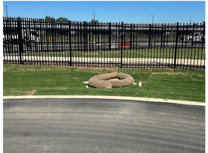
Photo 12: Permanent fencing, turf and sediment control
