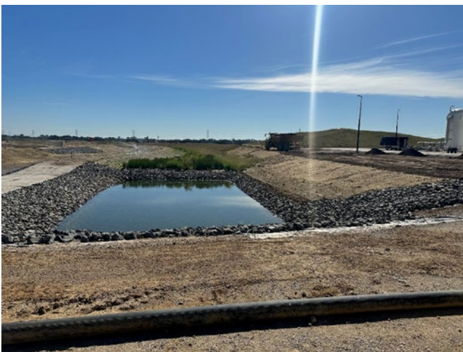
Photo 9: Water quality control pond, AWRC Outlet
