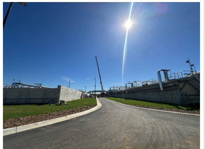
Photo 10: Completed internal roadway
