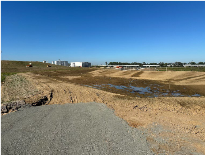
Photo 7: Operational bioretention basin
