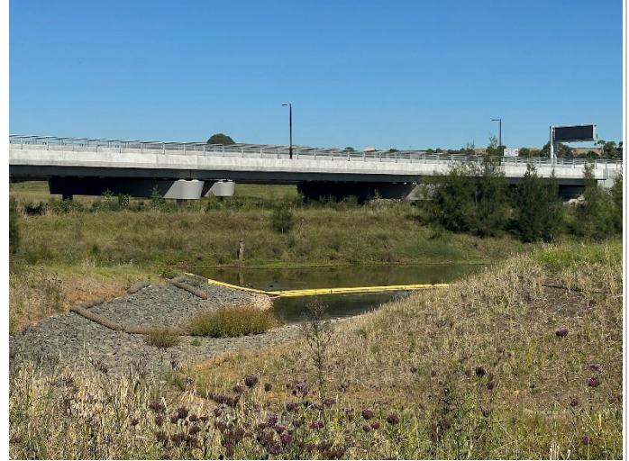
Photo 8: Silt boom within South Ck, downstream of emergency overflow channel
