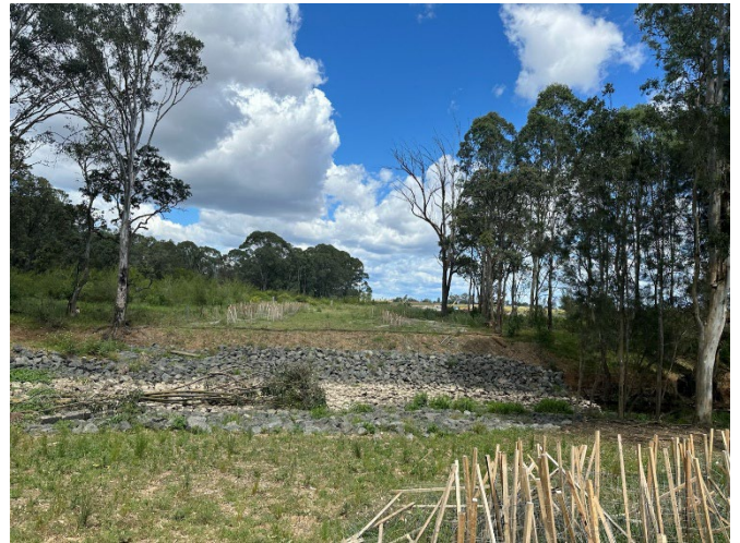
Photo 34: South creek rock scour protection
