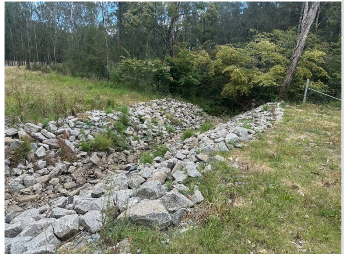
Photo 30: Creek crossing – scour protection
