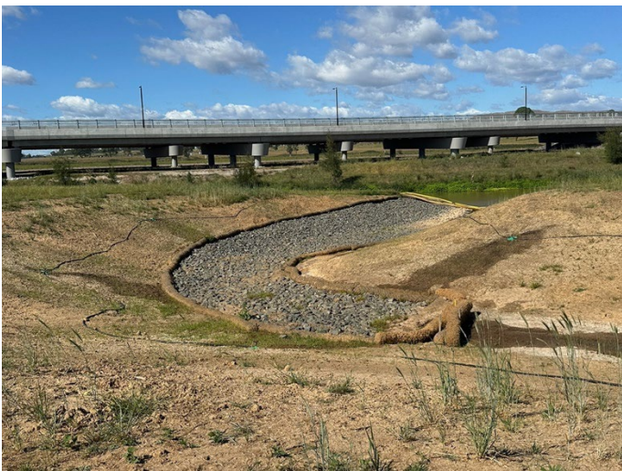
Photo 23: Permanent Rock scour protection
