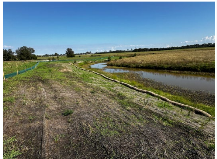
Photo 16: Jute mesh erosion control and creek protection
