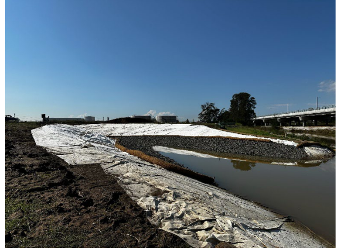
Photo 20: AWRC overflow outlet bank stabilisation works
