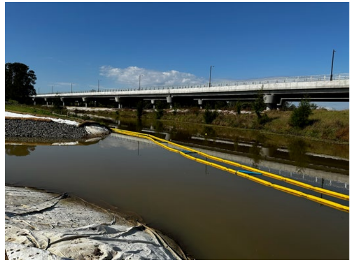
Photo 22: South Creek oil and sediment boom
