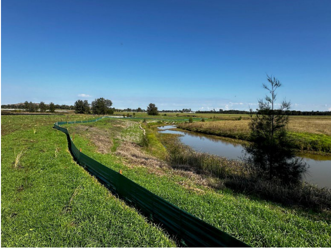
Photo 19: South creek embankment stabilisation and fauna fence
