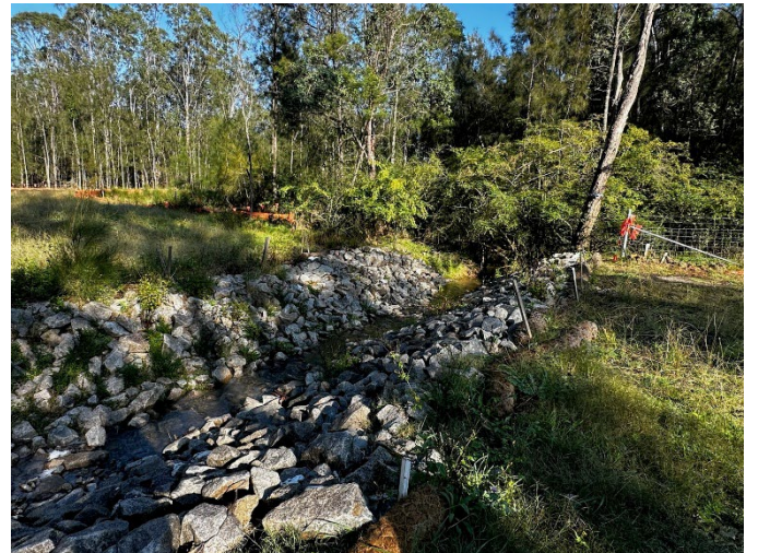
Photo 26: Permanent stream bank and scour protection
