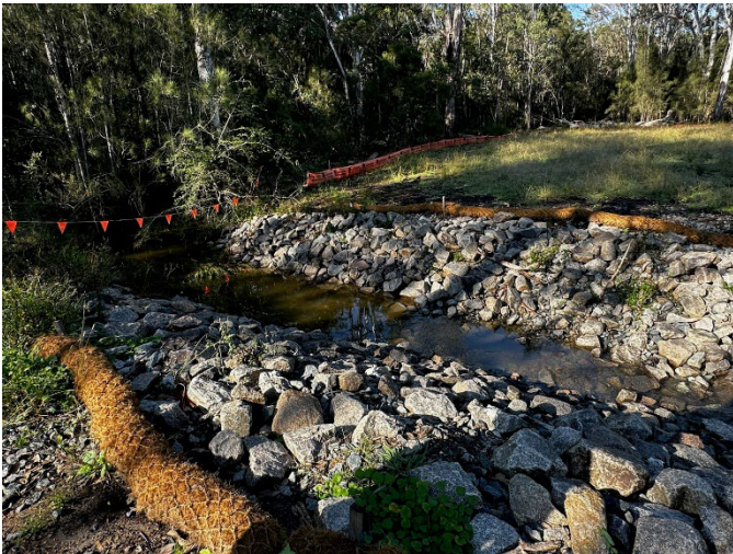
Photo 25: Permanent stream bank and scour protection
