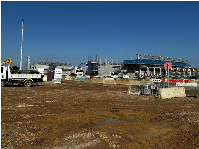
Photo 1: Sludge thickening and polymer storage units undergoing construction
