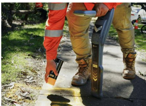
Service locating wand and spray paint marking
