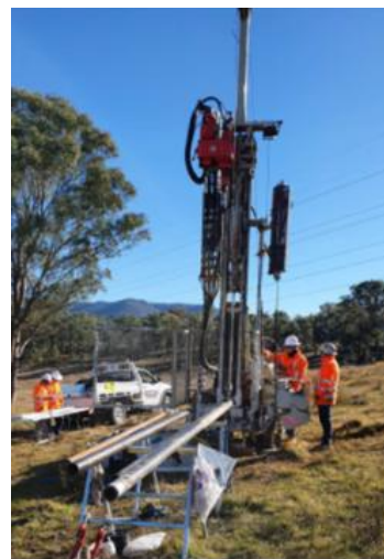
Typical drill rig for drilling boreholes
