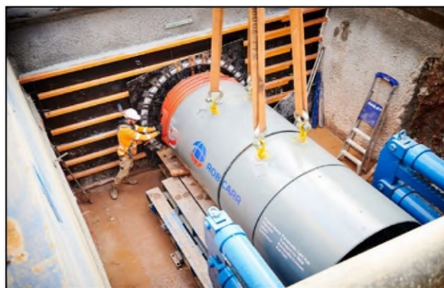
Example of a small tunnel boring machine. A similar machine which will be used for the Thornleigh Pipeline Duplication.
