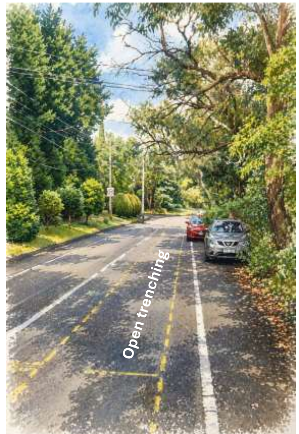
Figure 1 dotted lines painted on road to show approximate trench location and width.
