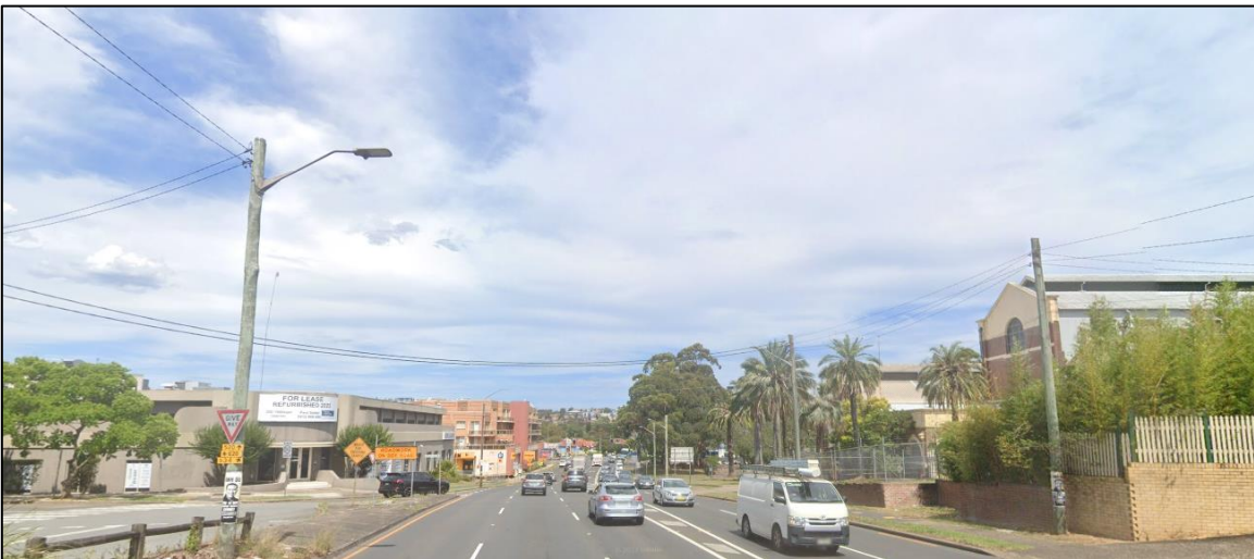
Figure 3-2: View east along Victoria Road at the Ryde Pumping Station frontage. (Source: Street View)
