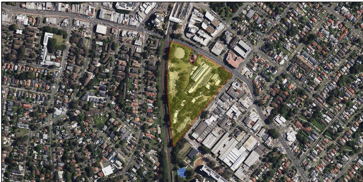
Figure 1-1: Aerial image of the Ryde Pumping Station (Source: SIXMaps)
