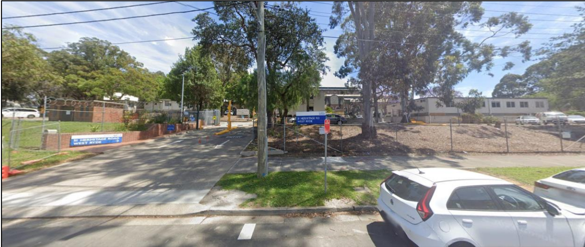
Figure 3-3: Frontage of Ryde Pumping Station along Hermitage Road, looking west. (Source: Google Street View)
