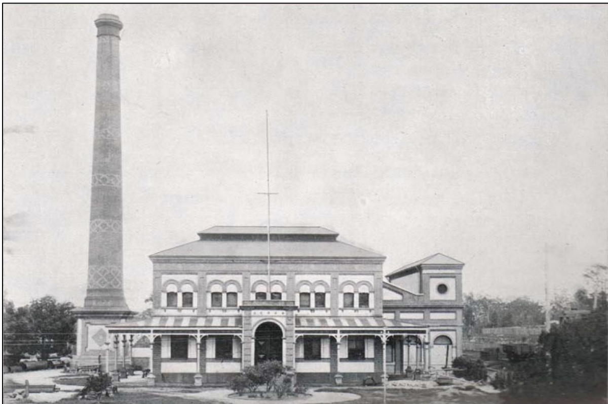
Figure 2-2: Photograph of the No. 1 Pumping Station, taken circa 1913. (Source: Sydney Water)
