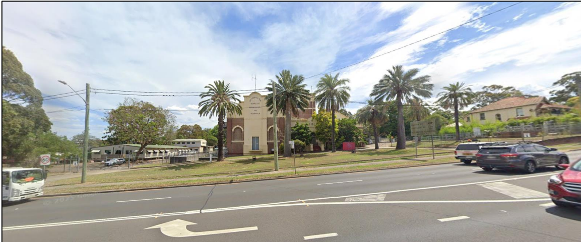
Figure 3-1: Ryde Pumping Station from Victoria Road, looking southwest (Source: Street View)
