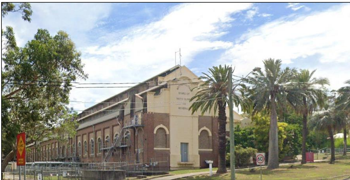
Figure 3-5: View of the northern frontage of the Ryde Pumping Station Engine House, facing southwest. (Source: Google Street View)
