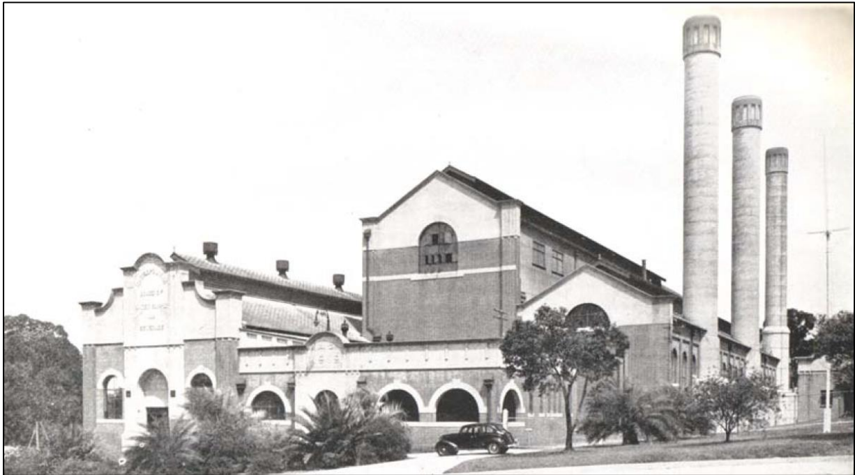
Figure 2-5: Photograph of the No. 2 Pumping Station, taken in 1939. (Source: Sydney Water)
