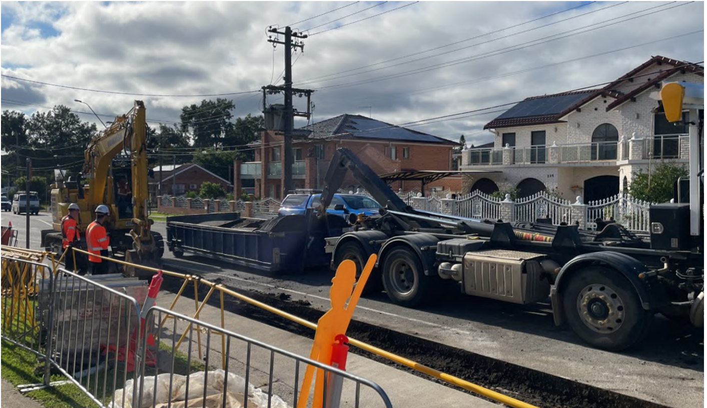
Figure 3-8 Trenched pipeline construction within road
