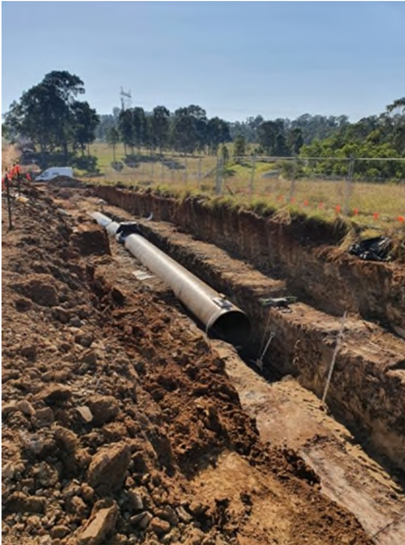
Figure 3-9 Trenched pipeline construction with benching
