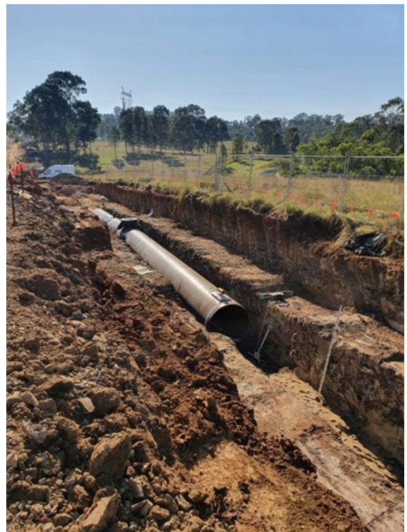
Image 4.2 Trenched pipeline construction with benching
