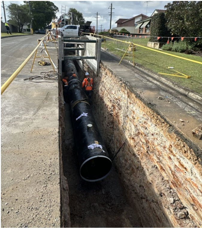
Image 4.1 Trenched pipeline construction within road
