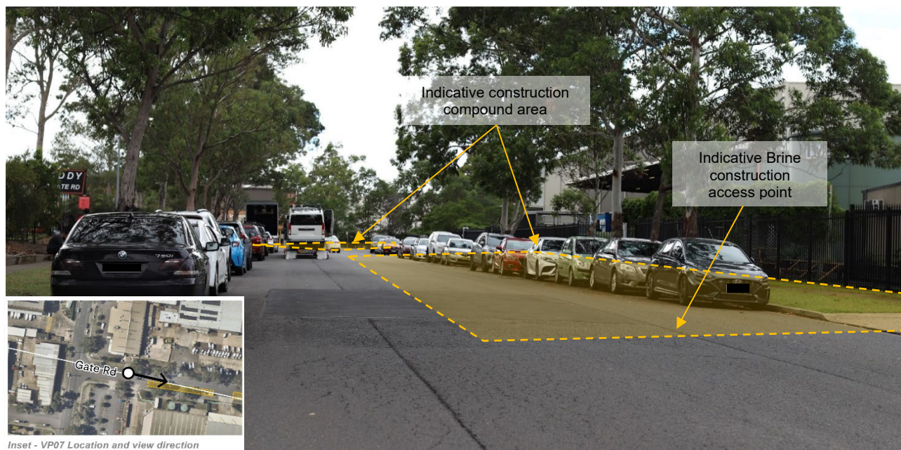
Figure 7.9 VP07 – View east on Gate Road showing construction compounds
