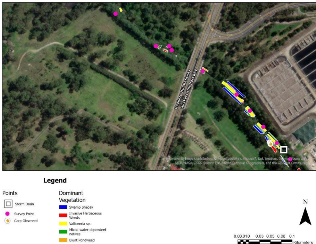
Figure 4-19 Survey points and dominant vegetation in Breakfast Creek from the WRRF to Quakers Hill Parkway
