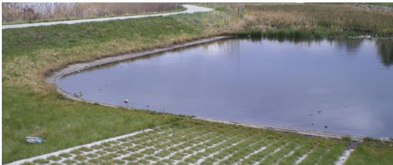
Figure 8-9 Example of a water quality basin
