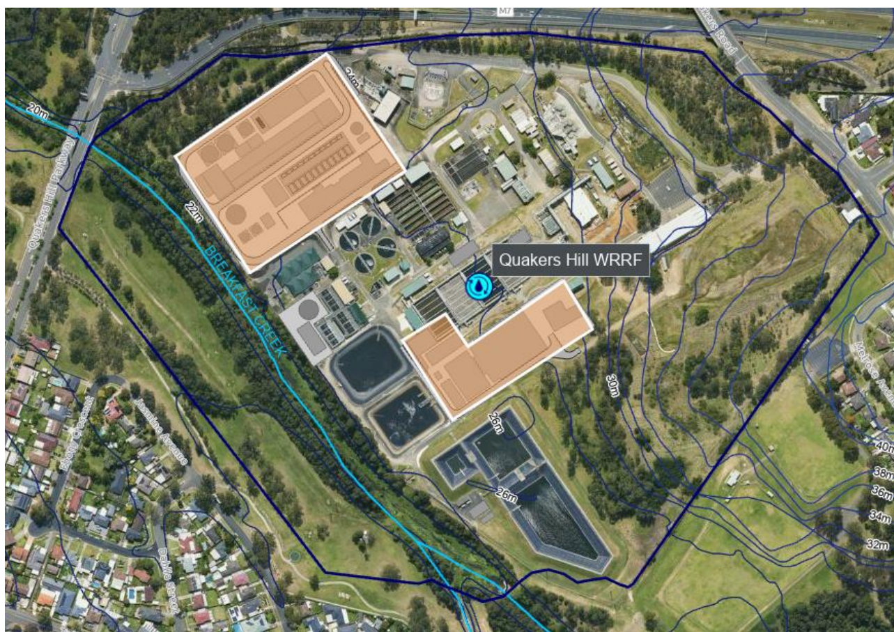
Figure 8-5 Advanced water treatment plant and secondary treatment system at Quakers Hill WRRF
