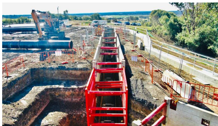
Pipes being installed at the Oran Park reservoir site
