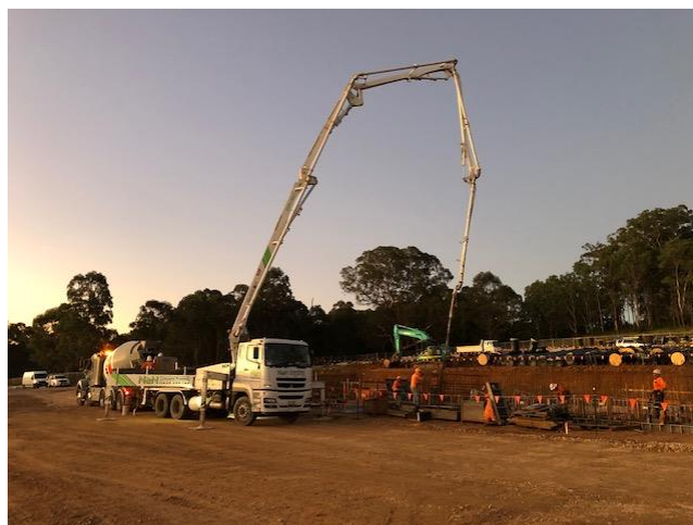
Concrete pour at Harrington Park pumping station.
