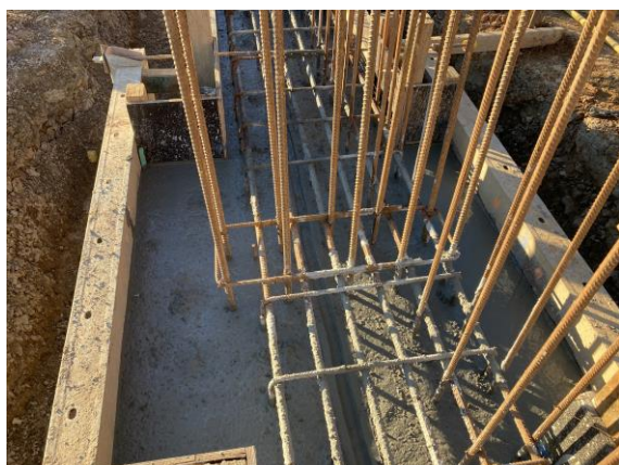
Steel form work set into the concrete foundation.
