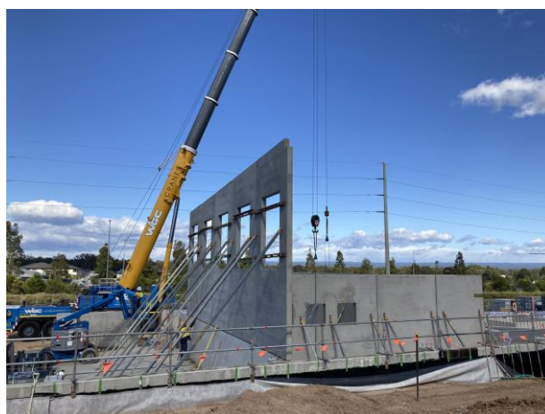
Pre-cast panels being individually lifted into place using a crane.
