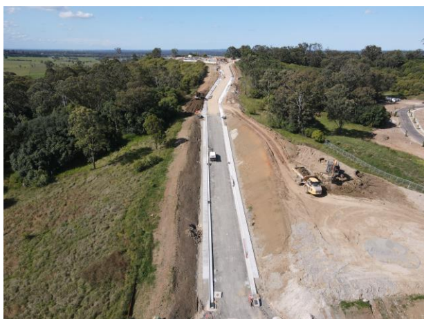
Civil works on the southern access road, including stormwater drainage, constructing kerb and laying asphalt.
