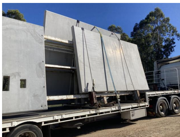
Pre-cast concrete panels being transported into site to form sections of the pumping station walls.
