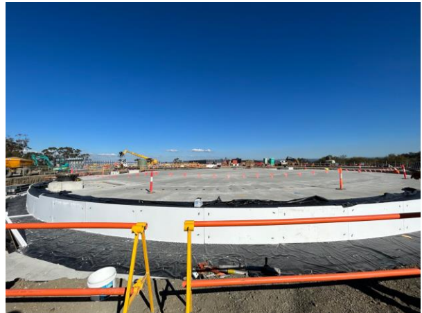
One reservoir base after a concrete pour. When construction is complete, each reservoir will hold 24ML of clean drinking water for Sydney Water customers across South West Sydney.
