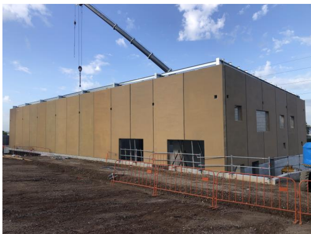
Installing more than 40 pre-cast panels to form the pumping station exterior. Each panel weighs up to 10T each!
