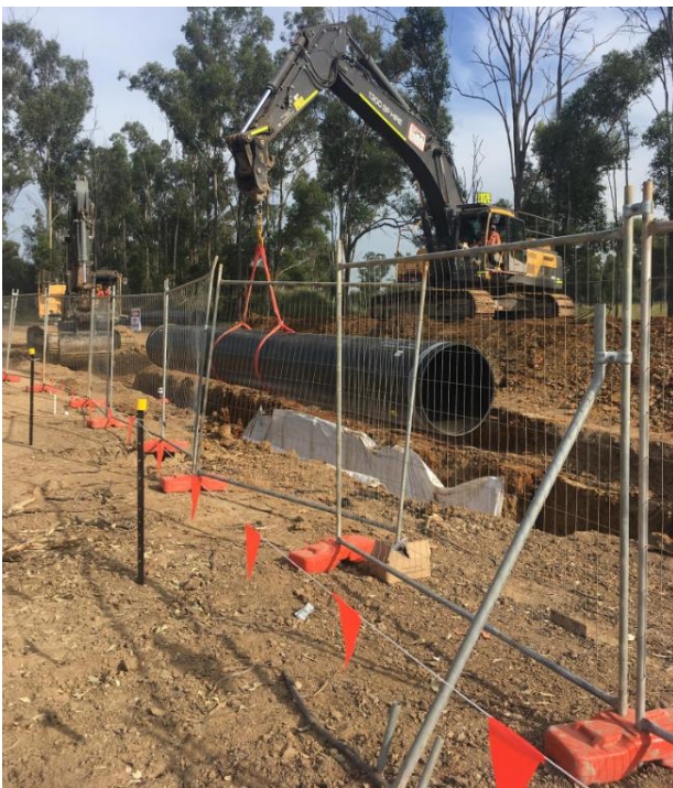
A section of water pipeline being lifted into place in Cecil Park.
