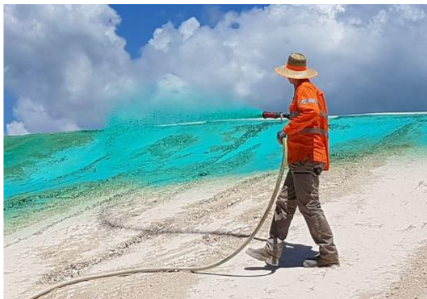
An example of an area that has been treated with a soil binding agent.
