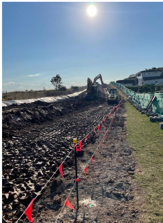
Backfilling the pipeline trench in William Howe.
