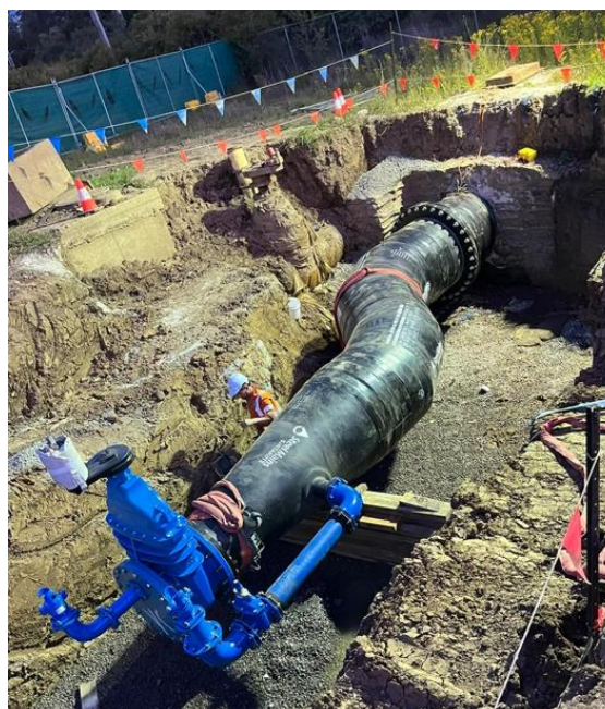
Connecting the new water main to the network inside The Australian Botanic Garden.
