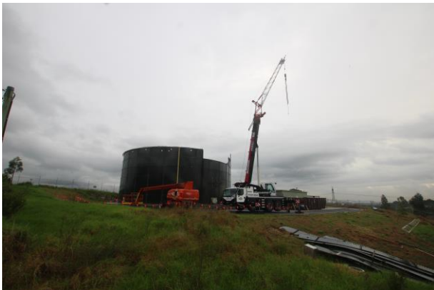
Demolition of old the Currans Hill Reservoir, removed panel by panel using a crane.
