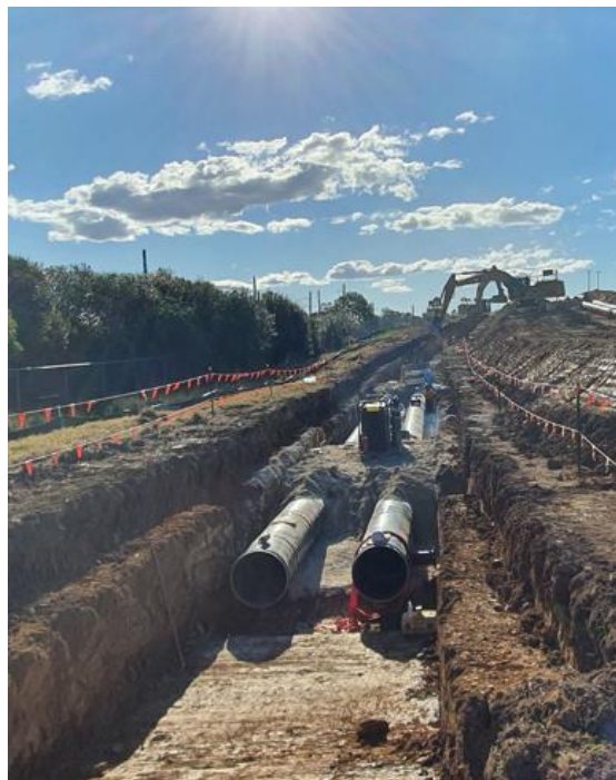
Twin pipeline installation inside The Australian Botanic Garden.
