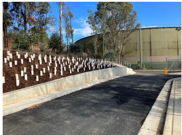
Completed landscaping, internal road, drainage and kerb to enable routine deliveries and maintenance checks by Sydney Water once the re-chlorination plant is operational.
