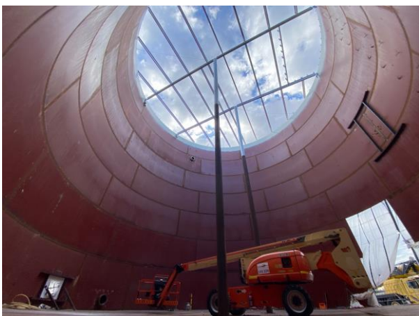
Interior view of the new Currans Hill Reservoir in preparation for painting, blasting and installation of the roof.
