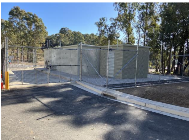
Completed installation of the re-chlorination plant which is currently being commissioned into operation.
