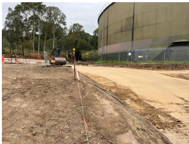
Compacting the internal access road at the Narellan South Reservoir using vibratory rollers and compaction equipment.
