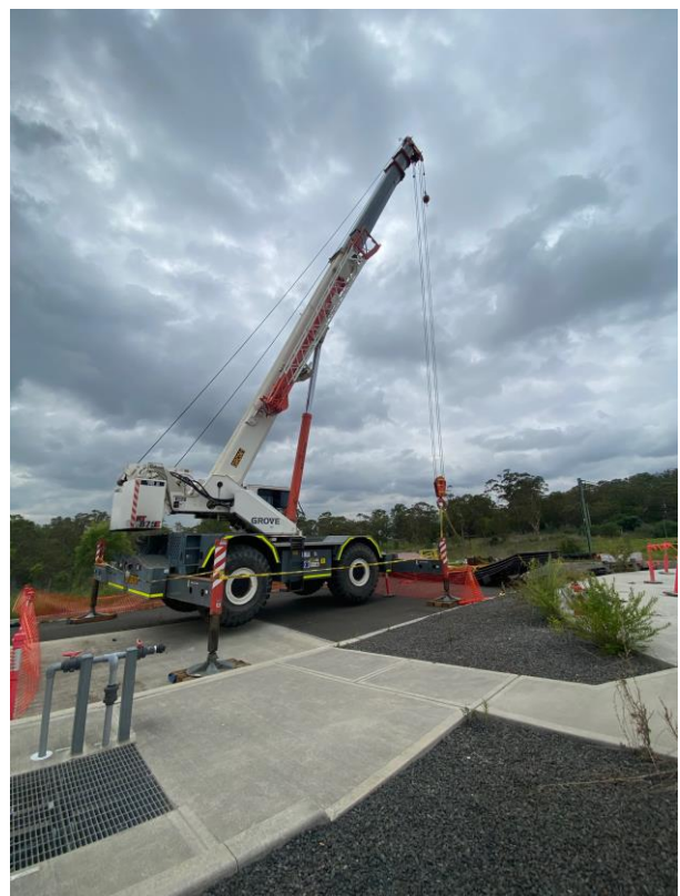
The crane at Currans Hill preparing to install steel plates weighing around 5 tonne each.
