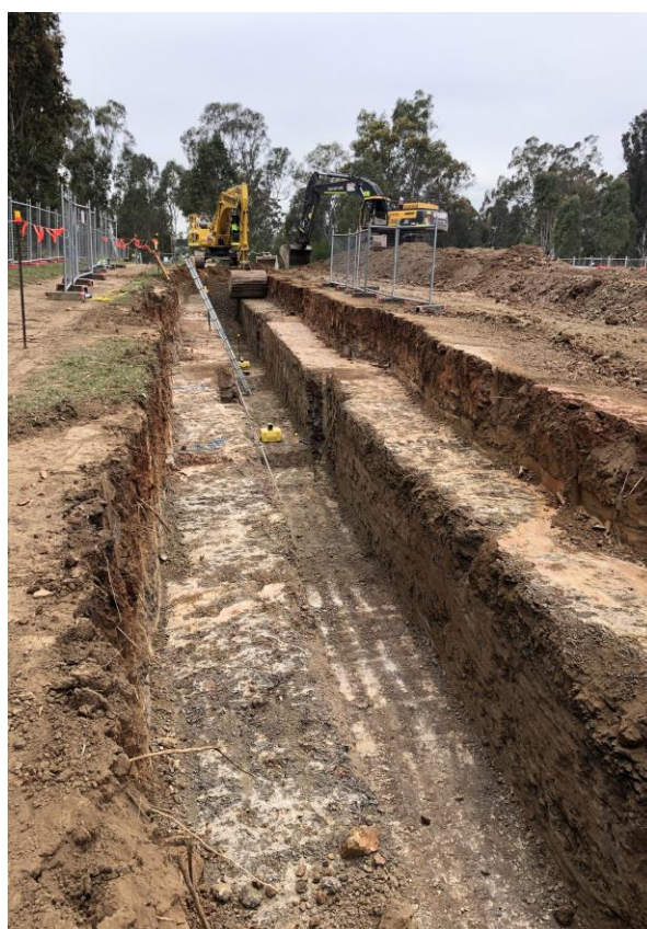
Construction of a new water pipeline at the Sydney International Shooting Centre in Cecil Park
