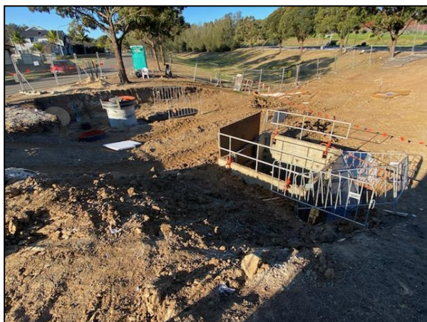
Work in the drainage reserve to install a scour pit.
