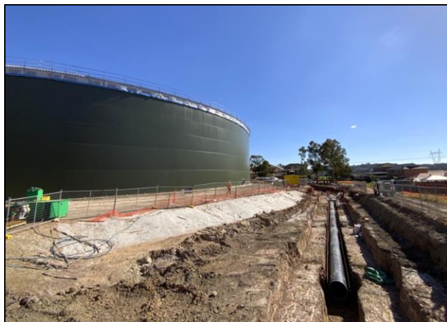
Pipework being installed next to the new reservoir.
