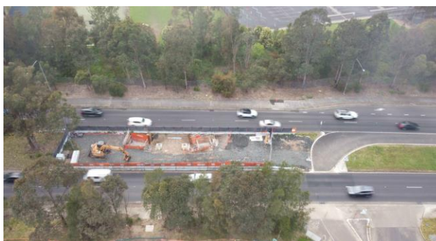
A view of a connection point between the new pumping station and existing Sydney Water network – located in the Cowpasture Road median.
