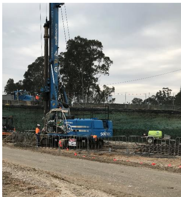
A rig installs piles for the new pumping station
