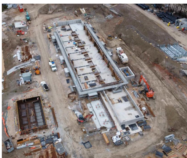
The Liverpool Reservoir pumping station sub-structure.
