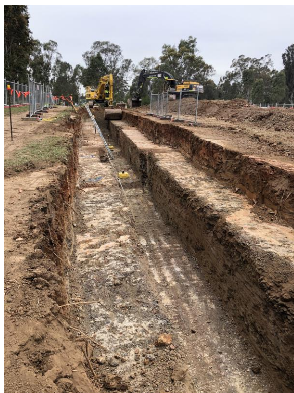
Construction of a new water pipeline at the Sydney International Shooting Centre in Cecil Park
