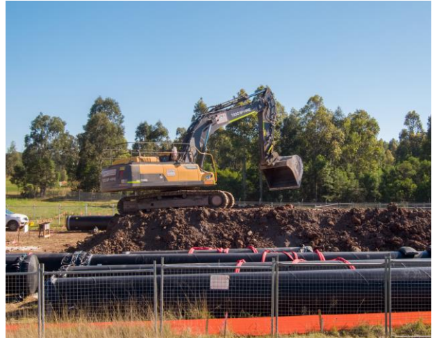
An excavator forms a stockpile as it digs a pipe trench
