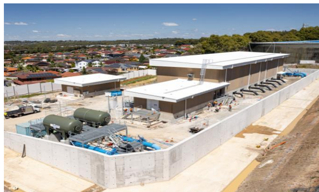
An aerial view of the completed retaining wall surrounding the new Pumping Station and high voltage switch rooms.
