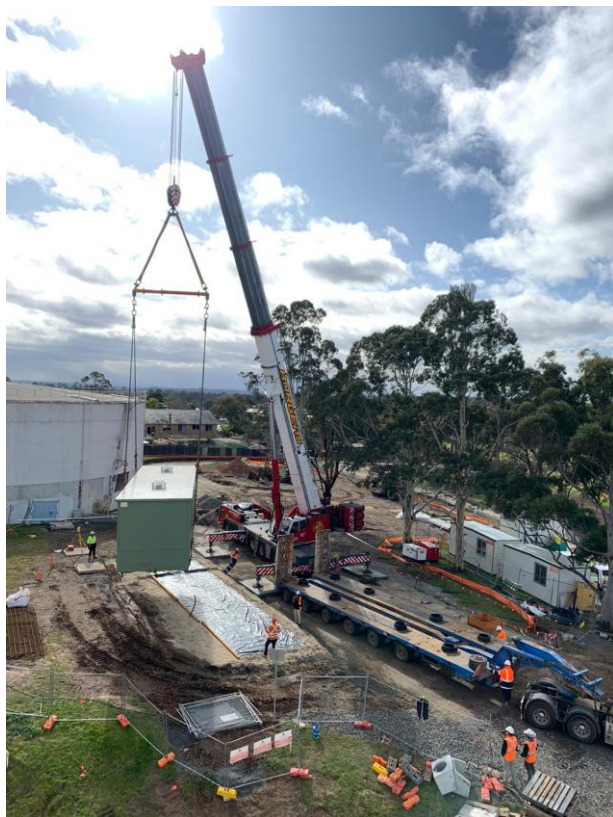
The new re-chlorination plant being lifted into position.
