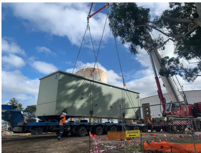
Moving the new re-chlorination plant during installation.
