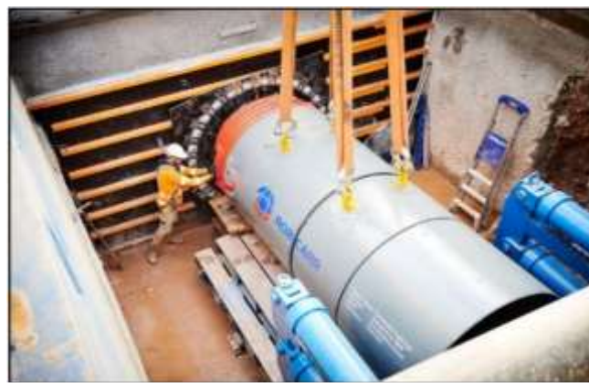
Example of a small tunnel boring machine, which will be used to create the tunnel.
