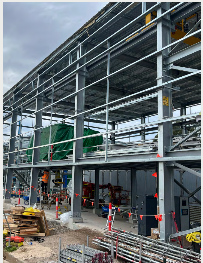
Carboniser dryer building under construction
