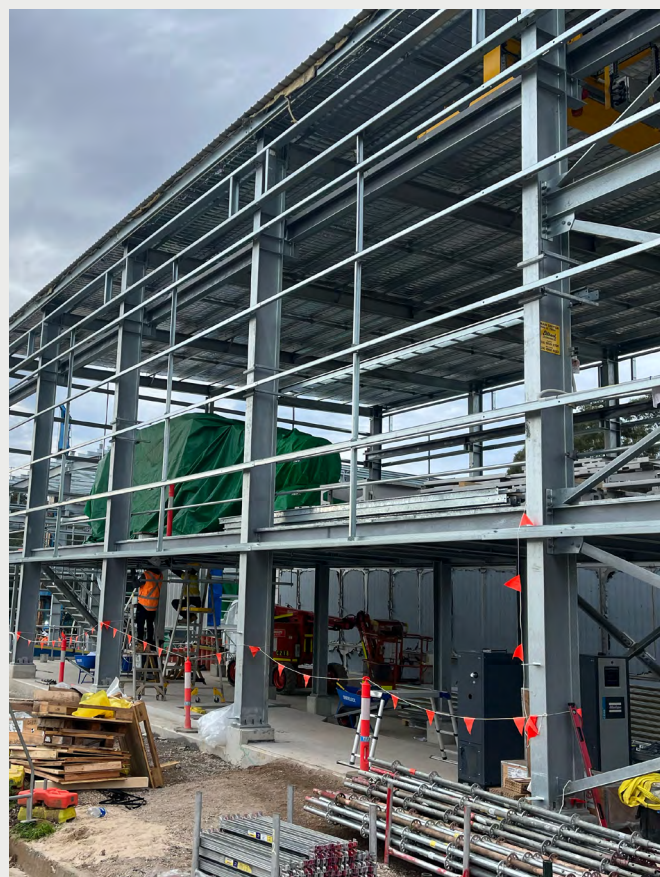
Carboniser dryer building under construction
