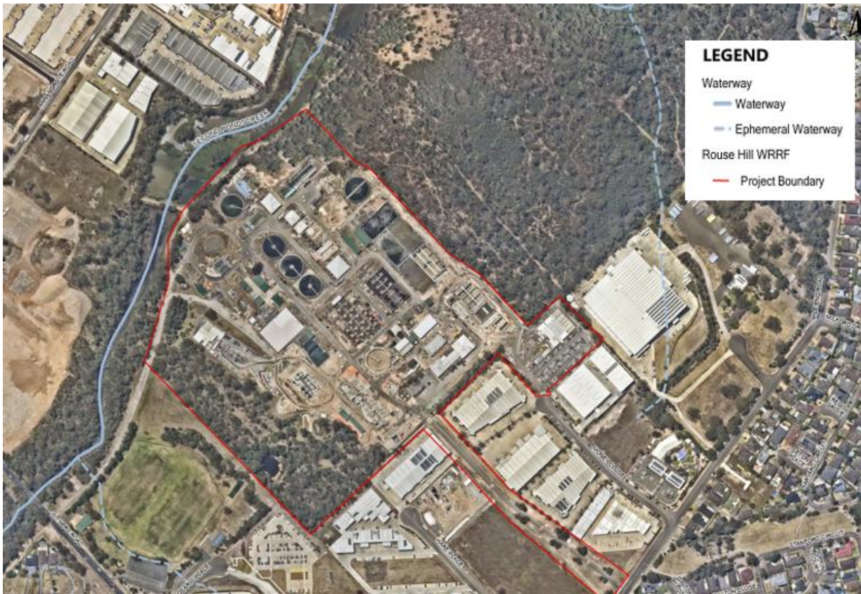
Figure 2 Rouse Hill WRRF in proximity to Second Ponds Creek
