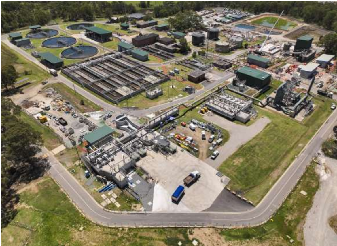
Figure 1: Riverstone Water Resource Recovery Facility
