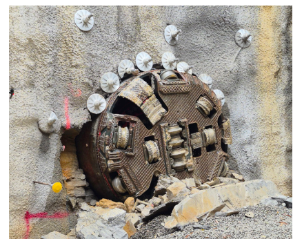
Tunnel Boring Machine breaks through at the pumping station, completing the tunnelling component of the North West Wastewater Connection.
