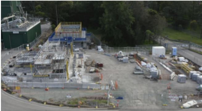
Switchroom site establishment and earthworks
