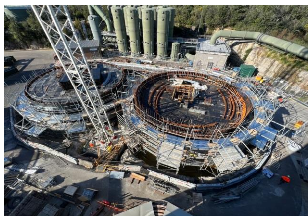
With the base of the digesters complete, our next step was to build the walls. The walls will be 15 metres high when finished, so we need to build them in three stages using a large tower crane.
