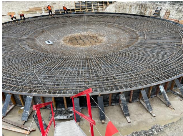
Our crew installing the steel formwork for the base of one of the two new digesters, ready for the concrete to be poured.
