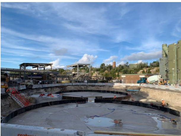
Our first step was to prepare the area for the two new digesters which involved relocating our cogeneration unit, some excavation, and early concrete work to form the foundation.
