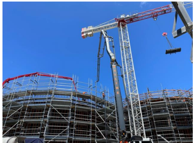
Our crew installing the steel formwork for the base of one of the two new digesters, ready for the concrete to be poured.
