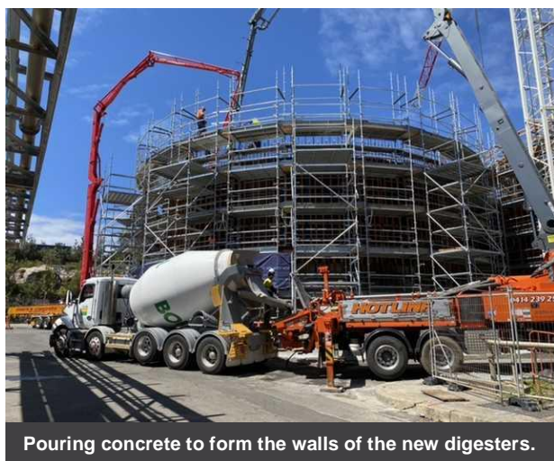
Our crew installing new formwork to build the walls of the new digester.
