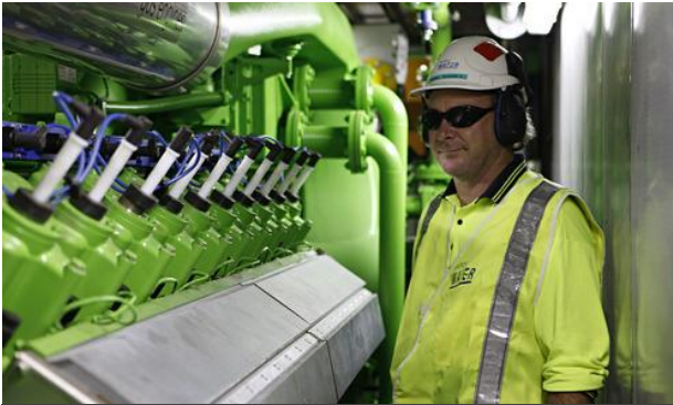
The cogeneration engine turns biogas into energy and heat.
