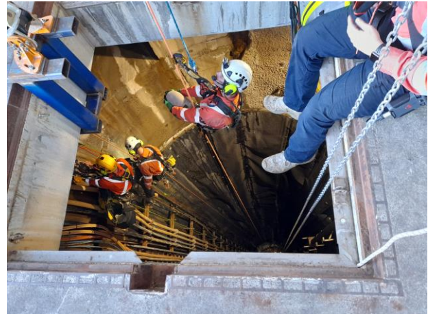
Our crew using specialised abseiling equipment to replace cabling that descends 160 metres below the surface
