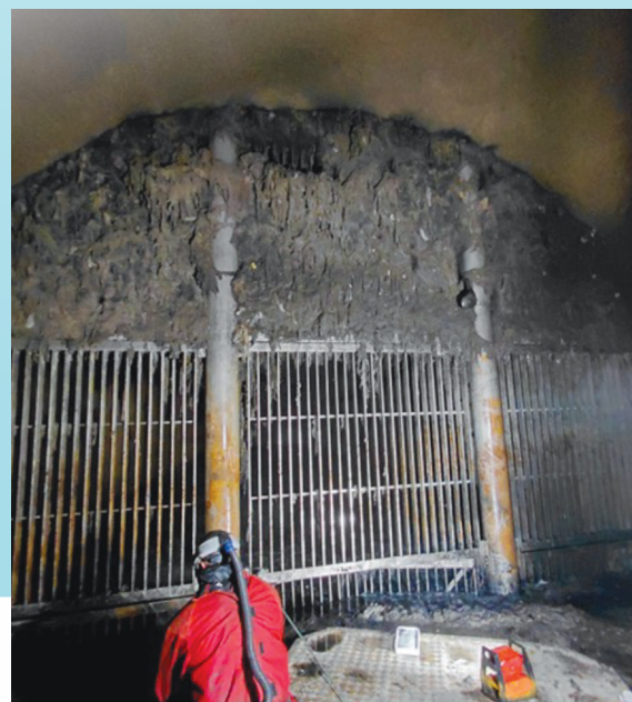
▲ Our workers deep underground at North Head cleaning rags, wet wipes and debris from the NST trash rack
