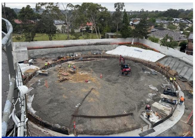
The view of our site from the top of the existing reservoir. We're finishing installing the tank foundation, which will support the new reservoir once it's built.
