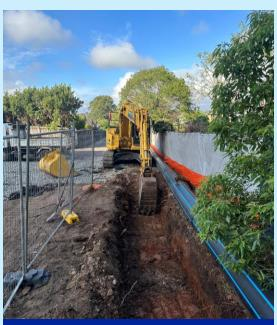
We excavated near our access road to install temporary pipes.
