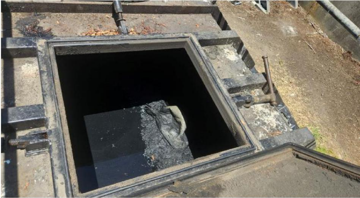
Figure 4: Decanting wastewater before moving silt off-site
