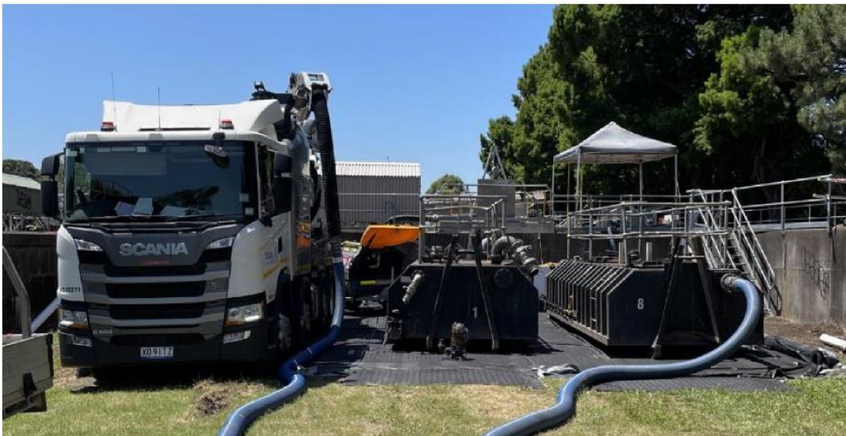
Figure 3: Site set-up for cross connection 2 Desilting
