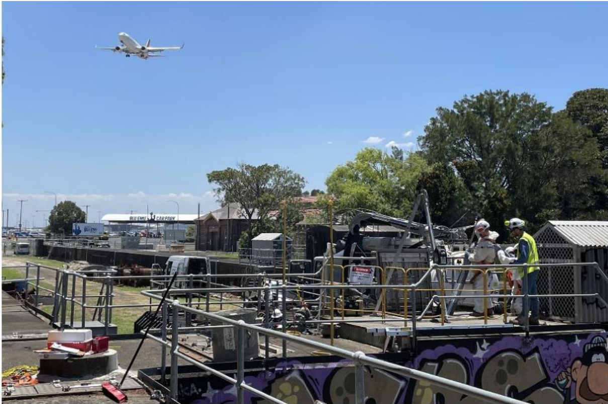
Figure 2: Desilting SWSOOS2 Package A1
