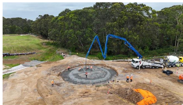
Half of the buffer tank, chamber base blinding concrete being poured
